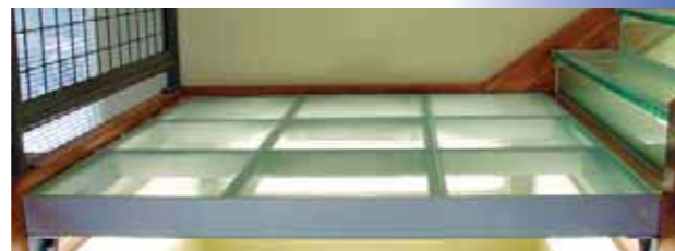
Total elapsed time for this stair landing: approximately 2 hours.
